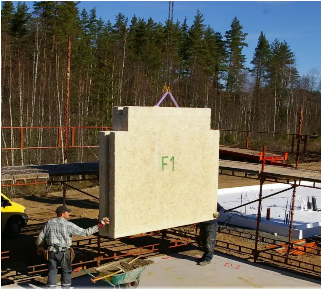
Step 3: Construct building using WWC – LWE systems
