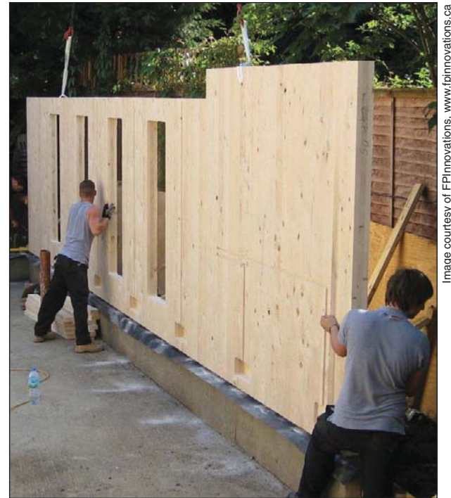
Installing a single cross-laminated timber wall panel.
